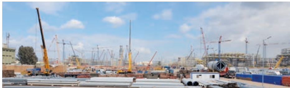
One of the largest investment projects currently in progress: the new refinery being built in Mostorod (Cairo)
