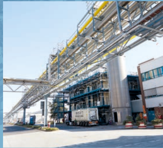
A total of 18 kilometres of pipe bridges and 300 kilometres of pipes can be found at Henkel's plant in Düsseldorf
