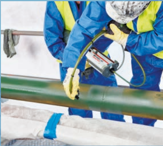
The final step of the Loctite® Composite Repair System is to apply several coats of Loctite® PC 7255 to protect the pipe against corrosion
