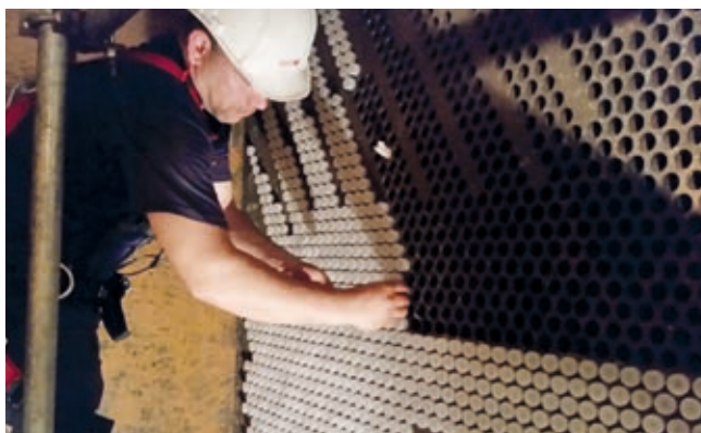
Plugs are first placed in the tubes before the tube sheet can be recoated
