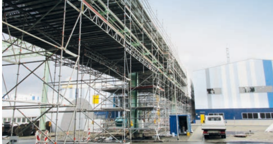
The 1,900m 2 steel structure, 800m 2 of piping, ca. 300 pipe supports and 750 pipe U bolts were coated in three separate phases
